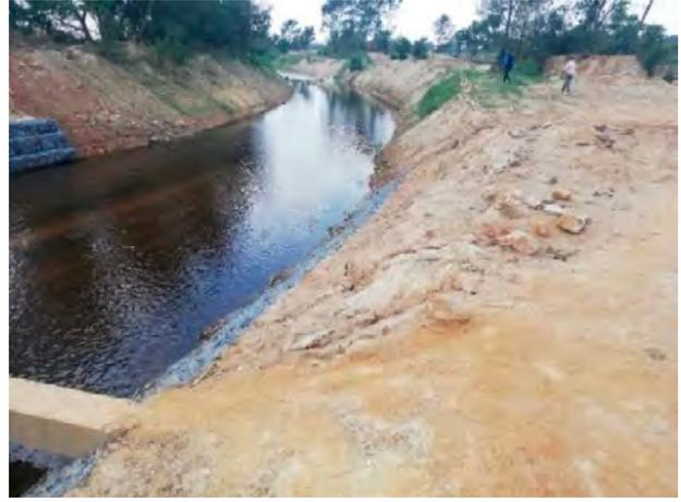
**Figure 22. Completed rehabilitation of the Van Ryn canal, with rediverted water**
