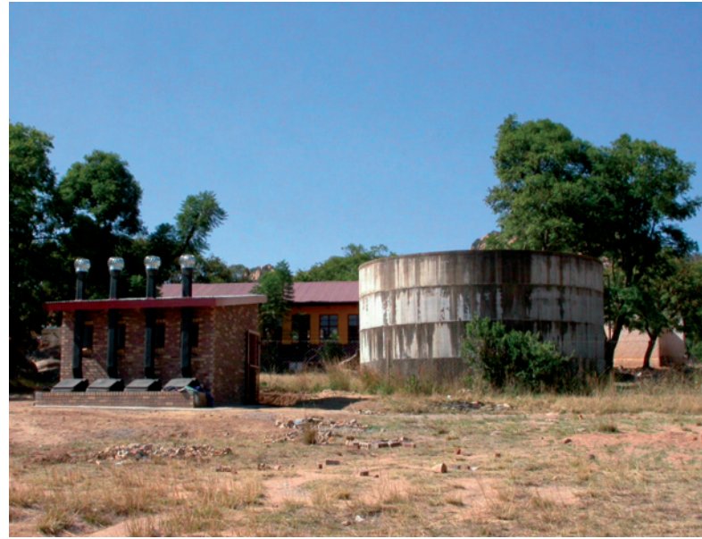
Pit latrines 8 m from a leaky concrete reservoir, GaMashashane.
