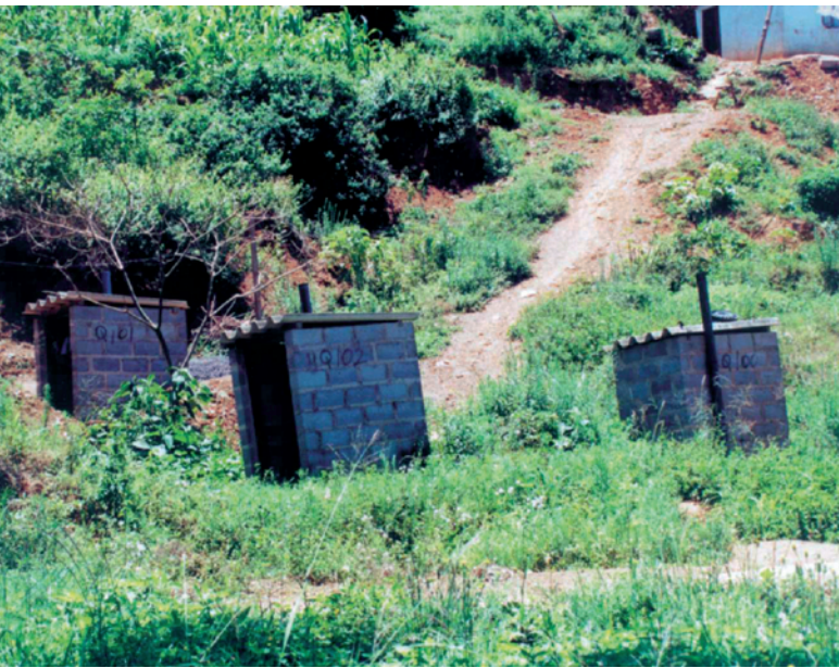
Sunken pit latrines in an area of collapsing soils in poorly drained landslide debris, Umlazi, Durban.
