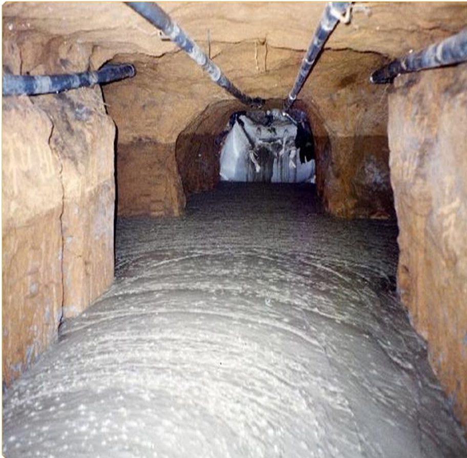
Cemented paste backfill underground.
