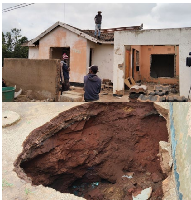
Figure 26: A small sinkhole causing damage to a house in Khutsong, Carletonville recorded in January 2025
