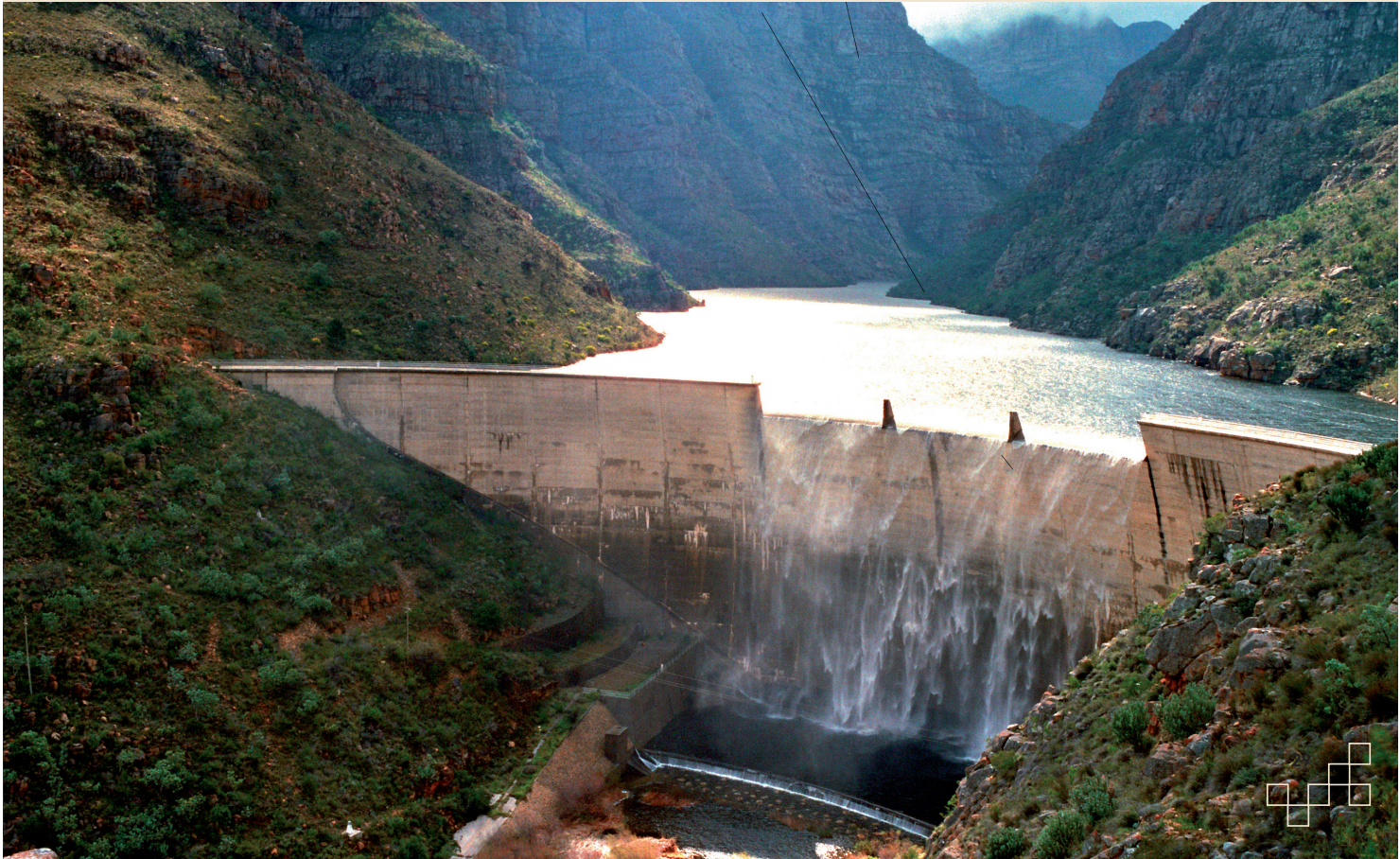
An engineering-geological appraisal for dam-safety purposes was conducted at the Roode Elsberg Dam, a 72-m-high double-curvature arch dam near Worcester.
