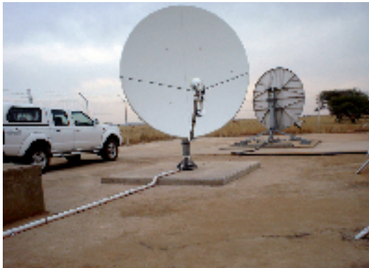
VSAT satellite dishes at the Central Recording Facility (CRF). The closest terminal transmits data in real time to the International Data Centre in Vienna.
