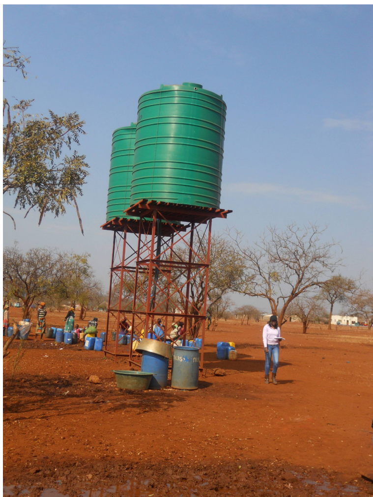
Borehole water storage reservoirs supplying communal taps at Ha-Nkomo village
