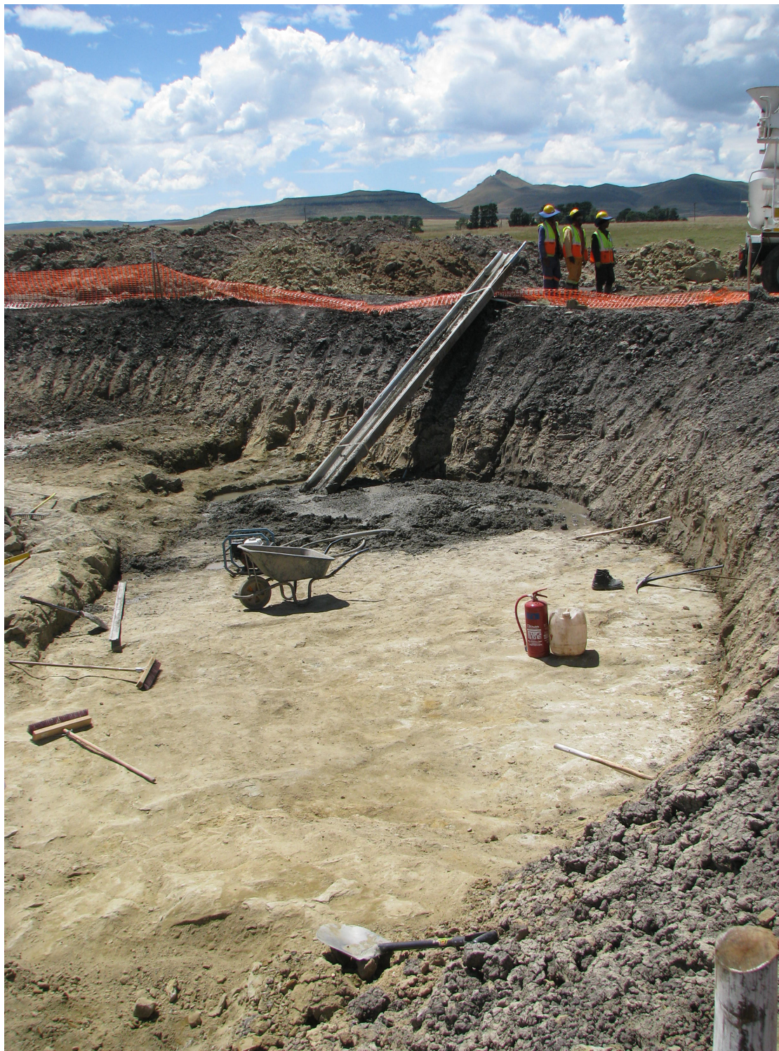
Classification of founding material at the Dorper Wind farm near Molteno in the Eastern Cape Province
